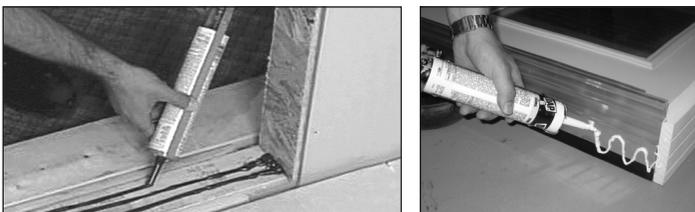
Variations in threshold designs may require that the caulk lines be applied directly to the bottom of the unit to ensure a weather-seal. Inspect the bottom of the sill for any flat surfaces or sill grooves. Apply caulk to sill bottom flat surfaces and grooves and also bottom of jambs. Apply a triple bead of caulk along sub-floor where unit will be positioned.
